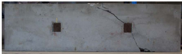
Fig. 11 Crack pattern for beam S05-80-3 [12]
