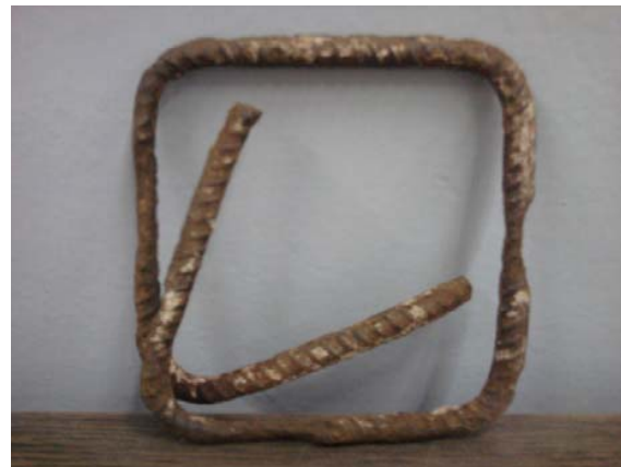
Fig. 7 Typical corroded column stirrup
