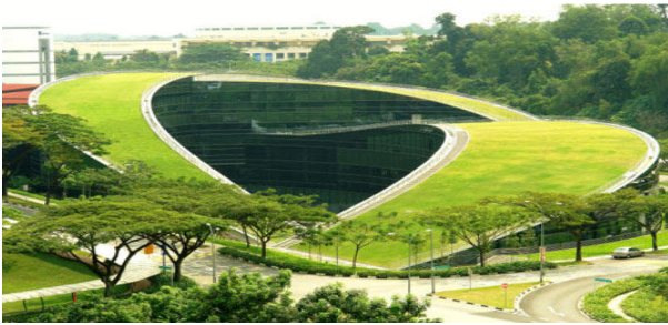
Fig. 4 Green roof on school of Art, Design and Media at Nanyang Technological University in Singapore
