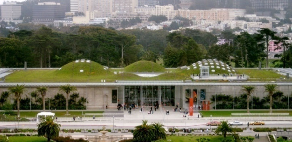
Fig. 3 Green roof on California Academy of Sciences [11]
