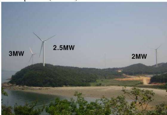
Fig. 4 YeungHeung wind test bed for domestic wind turbines.
