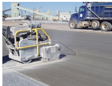
Fig. 3 Transvers joint
