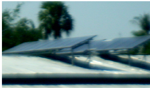
Fig. 5 PV Panel Installation on the roof of Building
