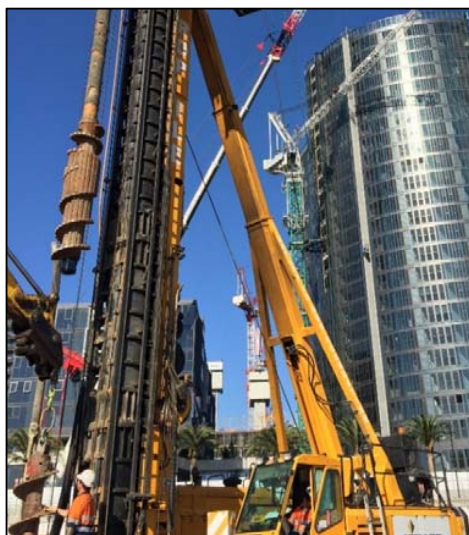
Fig. 7 Keller's modified DD drilling head
