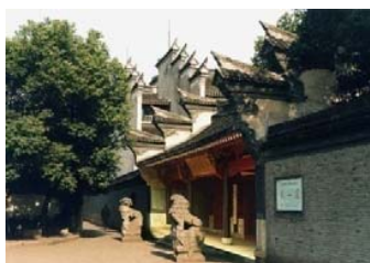
Fig. 3 The entrance to Tianyi Pavilion
