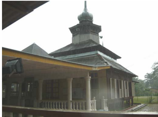
Fig. 2: Renovations and additional structure were supported to the Old Mosque of Ke. Mendun. in Negeri Sembilan.
