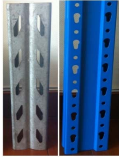
Fig. 1 Arrays of perforations of columns
