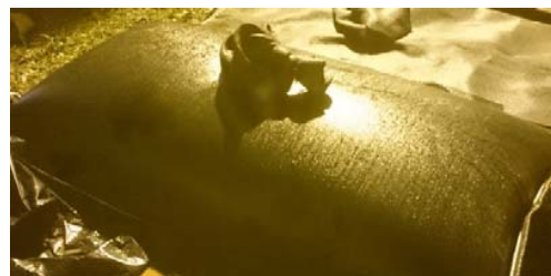
Fig. 3 Close geotextile system, geotextile tube
