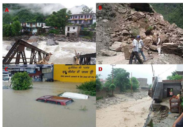
Fig. 2 A. Bridge collapsed due to flashfloods in Kanar village, Pithoragarh; B. Huge landslide on the Gangotri pilgrimage road; C. Roads are over flooded due to cloudburst-triggered floods in Dehradun city; D. Houses collapsed along the seasonal Nala in Kotdwar due to cloudburst (All these incidences occurred in the second week of August 2017)
