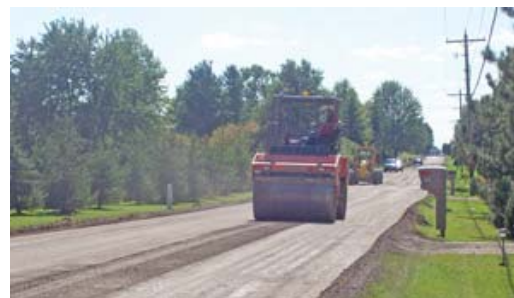
Fig. 3 Compaction of FDR base layer
