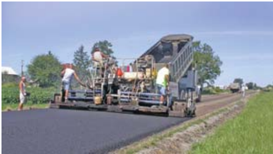
Fig.4 Resurfacing with hot mix asphalt
