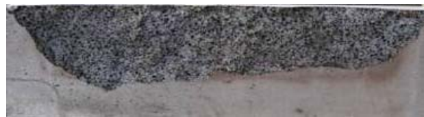
Fig. 4 State after testing – spalled concrete
