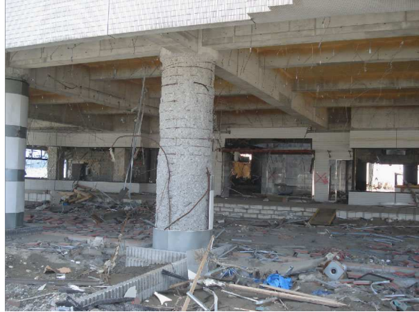
Fig. 20 Detail of RC columns
