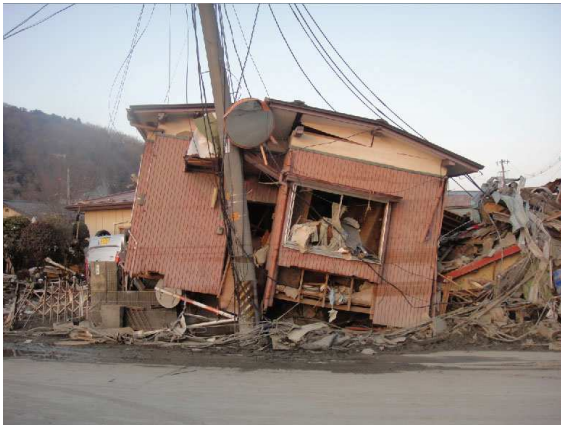
Fig. 9 Transportation of the upper floors
