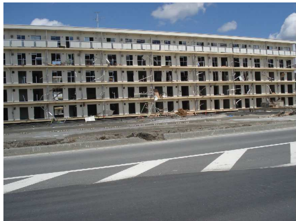
Fig. 17 Building at Rikusentakata city
