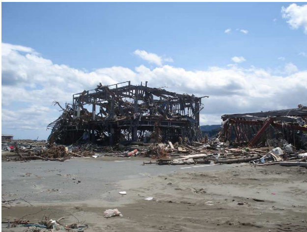
Fig. 14 Collapse of steel structure
