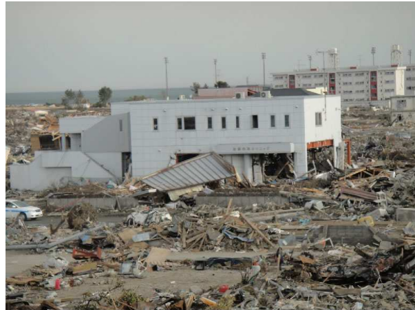
Fig. 11 Steel structure almost intact
