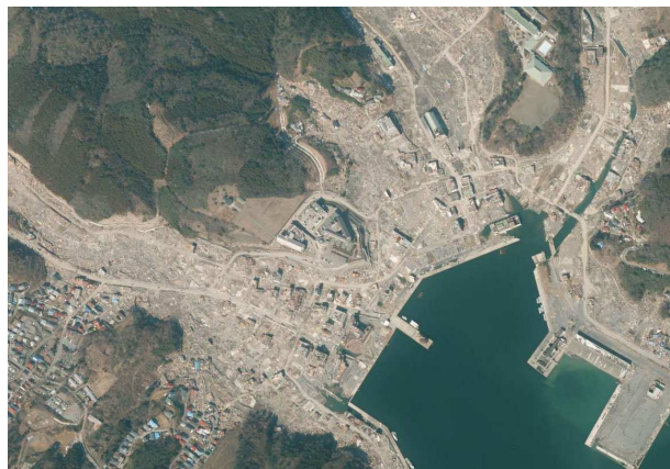
Fig. 5 Aerial view of Onagawa city after tsunami inundation
