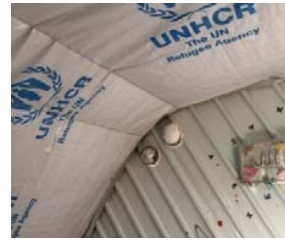
Fig. 17 Ventilation pipes closed [15]
