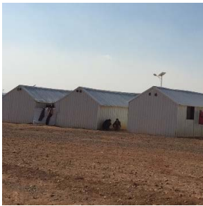
Fig. 21 Original gap between shelters [15]
