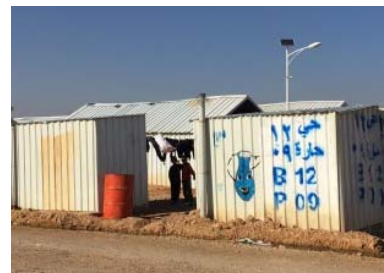
Fig. 19 Communal unit for toilet and shower [15]
