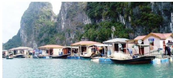
Fig. 3 Line of detached floating houses, Ha Long Bay, Vietnam [9]
