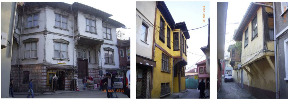
Fig. 11-13. The use of buttresses at the houses Photos: Özlem Köprülü Bağbancı, 2006
