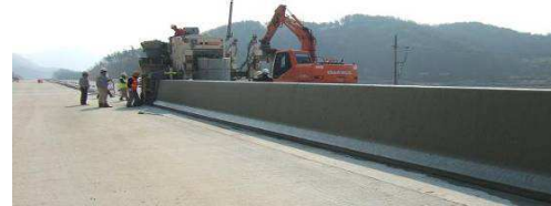
Fig. 1 Slipform Machine
