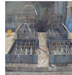
2. Installing Cast and Placing on Concrete Deck
