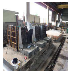
3. Installing Cast and Placing Concrete in Barrier
