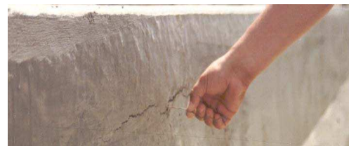
Fig. 2 Crack in Barrier
