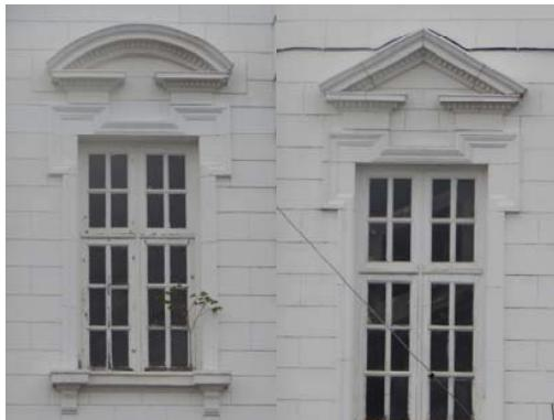
Fig. 23 (a) Circular and (b) triangular pediment as a window trim in Ipoh Railway Station
