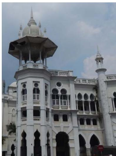
Fig. 17 Ground floor shows ogee arches, horseshoe arches and pointed horseshoe arches while the first floor shows double horseshoe arches and pointed horseshoe arches. At the roof top where there are dome chhatris which supported by multi-foil arches
