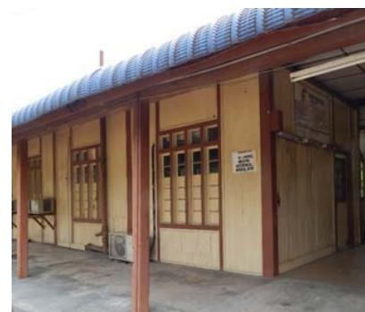
Fig. 21 The upper window part has been changed into glass to suit the usage of air-conditioned
