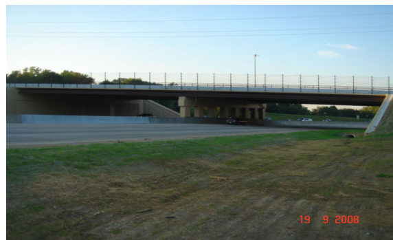
Fig. 1 Pacific Street and Interstate 680 Bridge, Omaha, Nebraska
