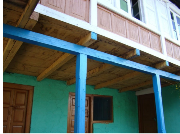
Fig. 6 Timber flooring and cantilevered balcony
