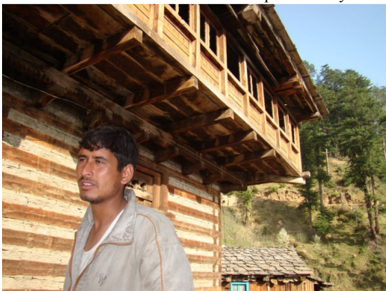
Fig. 5 Traditional 'Kath-khuni' wall construction with timber & stone
