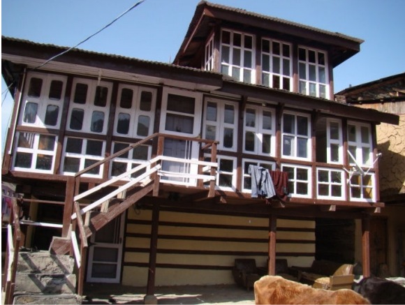
Fig. 8 Indigenously built "solarium" or "sun-space" created in dwellings
