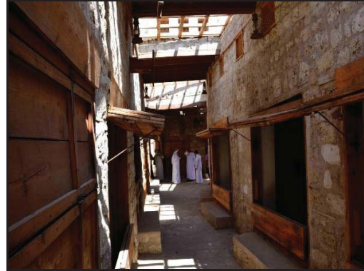
Fig. 4 Souq Al-Lail after being restored
