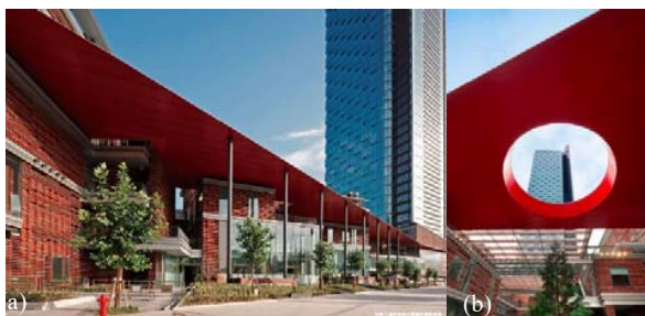
Fig. 4 (a) 200 m long cornice, (b) the hole in it
