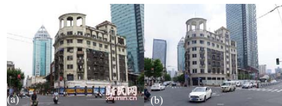
Fig. 5 (a) Photo of Hongkou Building from the intersection of North Sichuan Road and Haining Road before renovation taken on 2012, (b) after renovation taken on 2016
