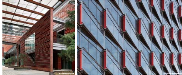
Fig. 10 (a) Clay pipe surface, (b) red surface of vents in high-rise office building
