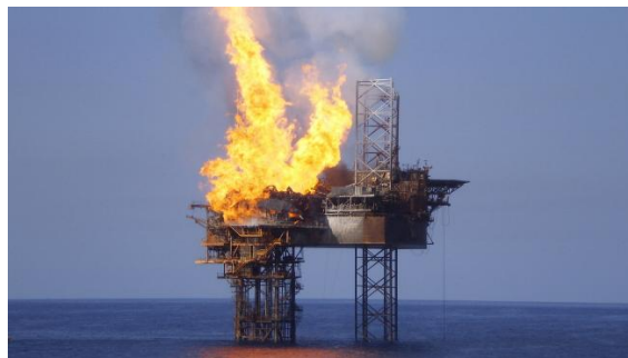
Fig. 2 A major platform fire [17]
