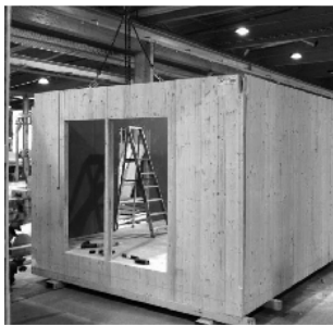
Fig. 6 Fabrication of CLT module elements
