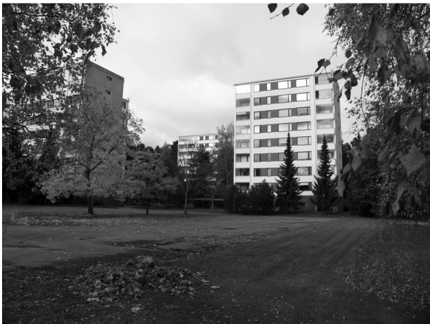
Fig. 1 A significant number of suburbs were constructed in Finland in the 1960's and 1970's
