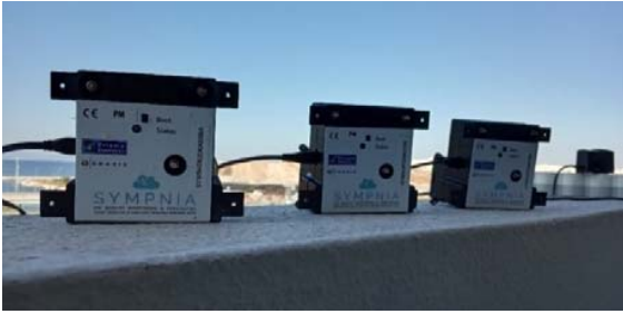
Fig. 6 Three different IoT platforms have been installed in the same location in order to proceed with sensitivity testing
