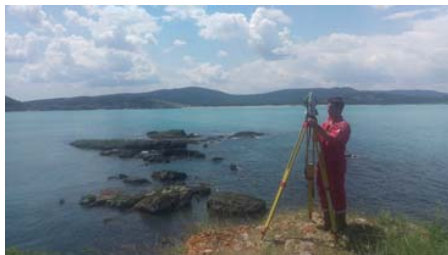
Fig. 8 Photograph showing the use of a Leica FlexLine TS06 plus to fix the static points of the trenches geographically (Photograph Michael Grant)
