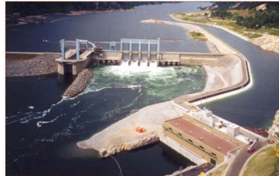
Run of river hydro plant
