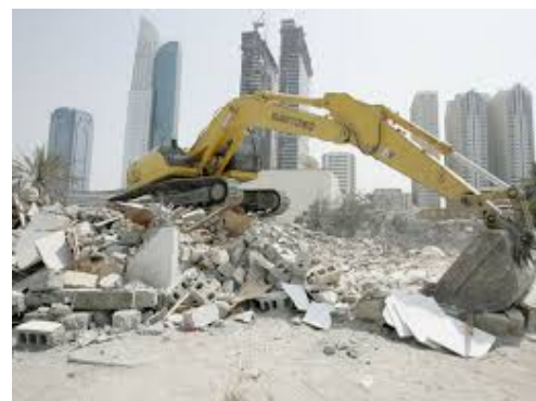
Fig. 3 Demolition of buildings [10]
