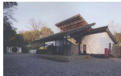
Fig. 6 The hip roof on the Square Pagoda Garden's north gate [10]
