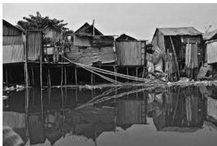
Fig. 5 Environmental condition of slum [35]
