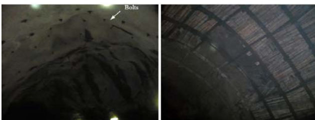
Fig. 2 Places with reinforced support in the ramp
