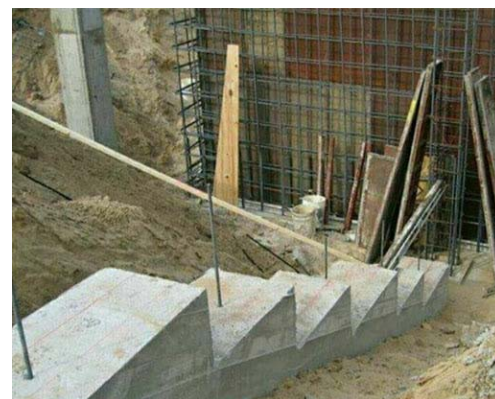
Fig. 1 Execution of stepped foundation in sloping lands
