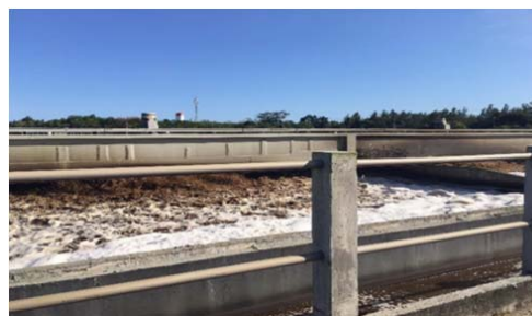
Fig. 1 Chemical effluent treatment station at CETREL
