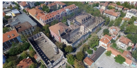
Fig. 9 The aftermath of the fire [16]
