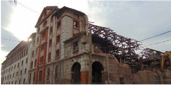
Fig. 7 The partially demolished tobacco warehouse [14]
