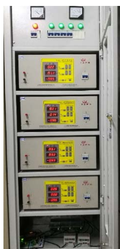
Fig. 5 Potentiostatic monitoring field photos
