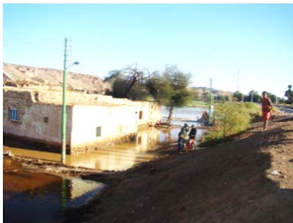
(a) Roads destroyed by flood waters
