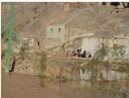
(b) Buildings destroyed by flood waters
