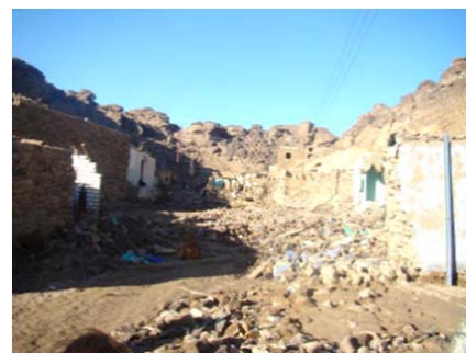
(b) Flood damaged urban areas
