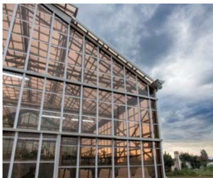
Fig. 8 100 m 2 greenhouse prototype made with DSSC solar panels
