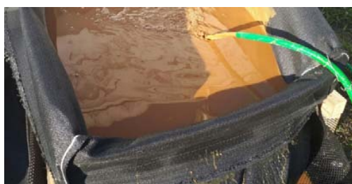
Fig. 2 Open geotextile system, drying bed
