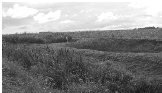
Fig. 3 Subsurface constructed wetland in the farm Mezaciruli, Latvia. Photo: Linda Grinberga
