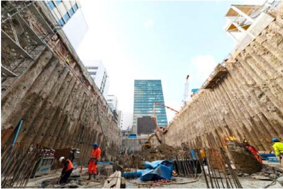
Fig. 3 View out of the excavation pit towards west
