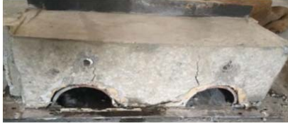
Fig. 4 First trial of concrete block
