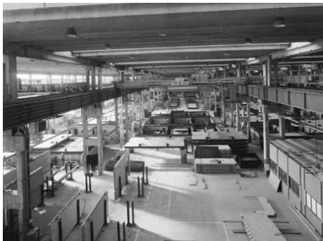
Fig. 2 Prefabricated sandwich panel factory in Hungary, 1974 [15]
