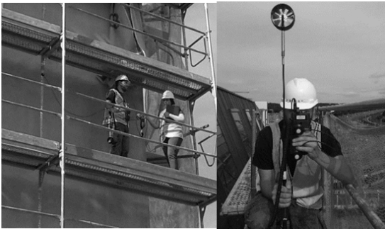
Fig. 1 The measurements on the scaffolding
