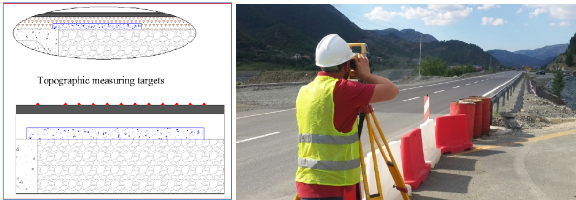
Fig. 4 Topographic field measurements
