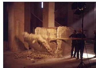
Fig. 5 Beirut National Museum. Rehabilitation after the civil war (1975-1991). Removing the cement box which covers a Roman Sarcophagus [4]
