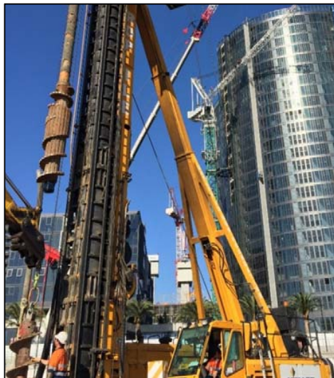
Fig. 7 Keller's modified DD drilling head
