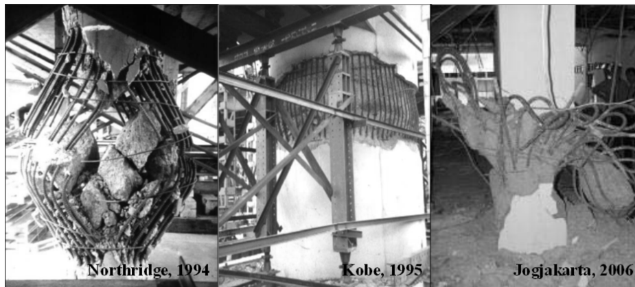
Fig. 1 The failure of structure in vertical earthquake
