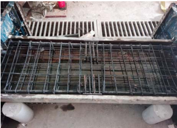
Fig. 4 Detail of reinforcement in deep beam
