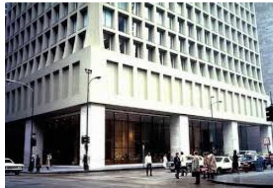
Fig. 2 Continuous deep beams supported on concrete columns
